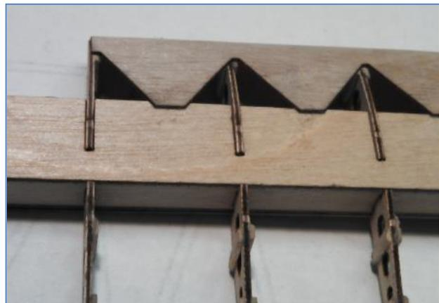
Figure 1.9 Leading Edge Gluing Detail
